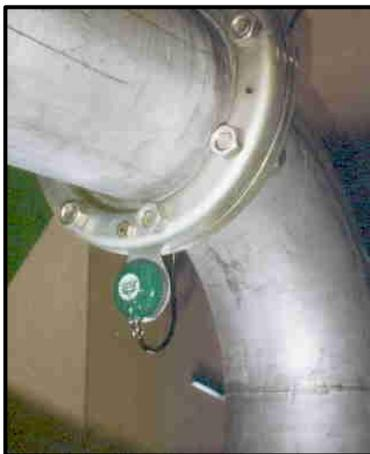
It is important that the sensor is sited correctly for each application. The sensor must be installed near to where the acoustic energy is being generated.
