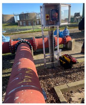
The DFM 6.1 Doppler Flow Meter transmits continuous high-frequency ultrasound through the pipe wall into the flowing liquid. Sound is reflected to the single sensor from suspended solids or gas in the liquid. If the liquid is flowing, the reflected sound returns at a shifted frequency, and the DFM 6.1 continuously measures this frequency shift to accurately measure velocity.
