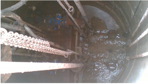
A typical wet well application where Quantum 2 is used for Pump Control.
