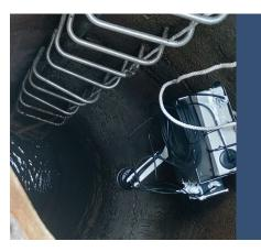
"By combining Pulsar Measurement's non-contacting dBi transducer range with the Taiwanese local NB-IoT system they could provide the low-power accurate level monitoring that the Sewerage Systems Office required."
